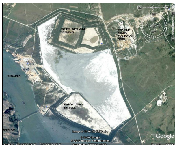
Fig. 2 - The waste heaps complex from Moldova Noua (Google Earth)
